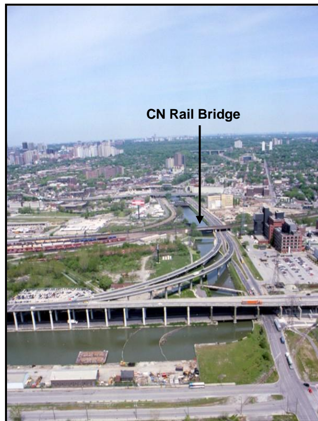
Figure 5-3 Location of CN Rail Bridge in the Project Study Area
